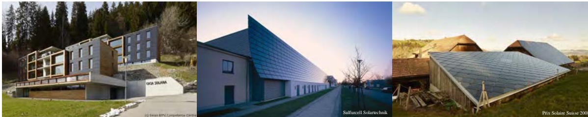
Source: Institute of Applied Sustainability to the Built Environment (ISAAC), Swiss BiPV Competence Centre Campus, Trevano CH-6952 Canobbio, www.bipv.ch
