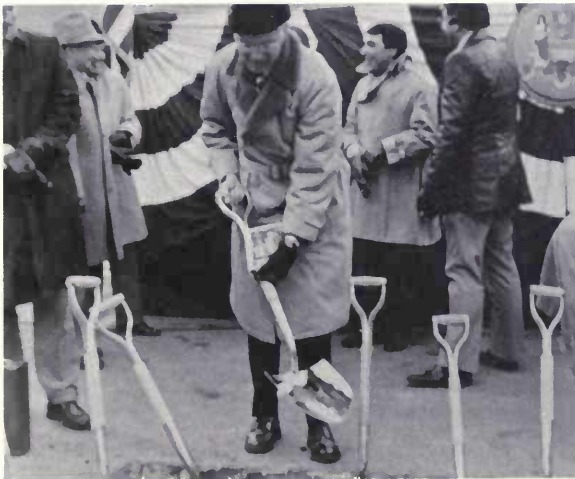
breaking ground for new Wills Eye Hospital c. 1978
