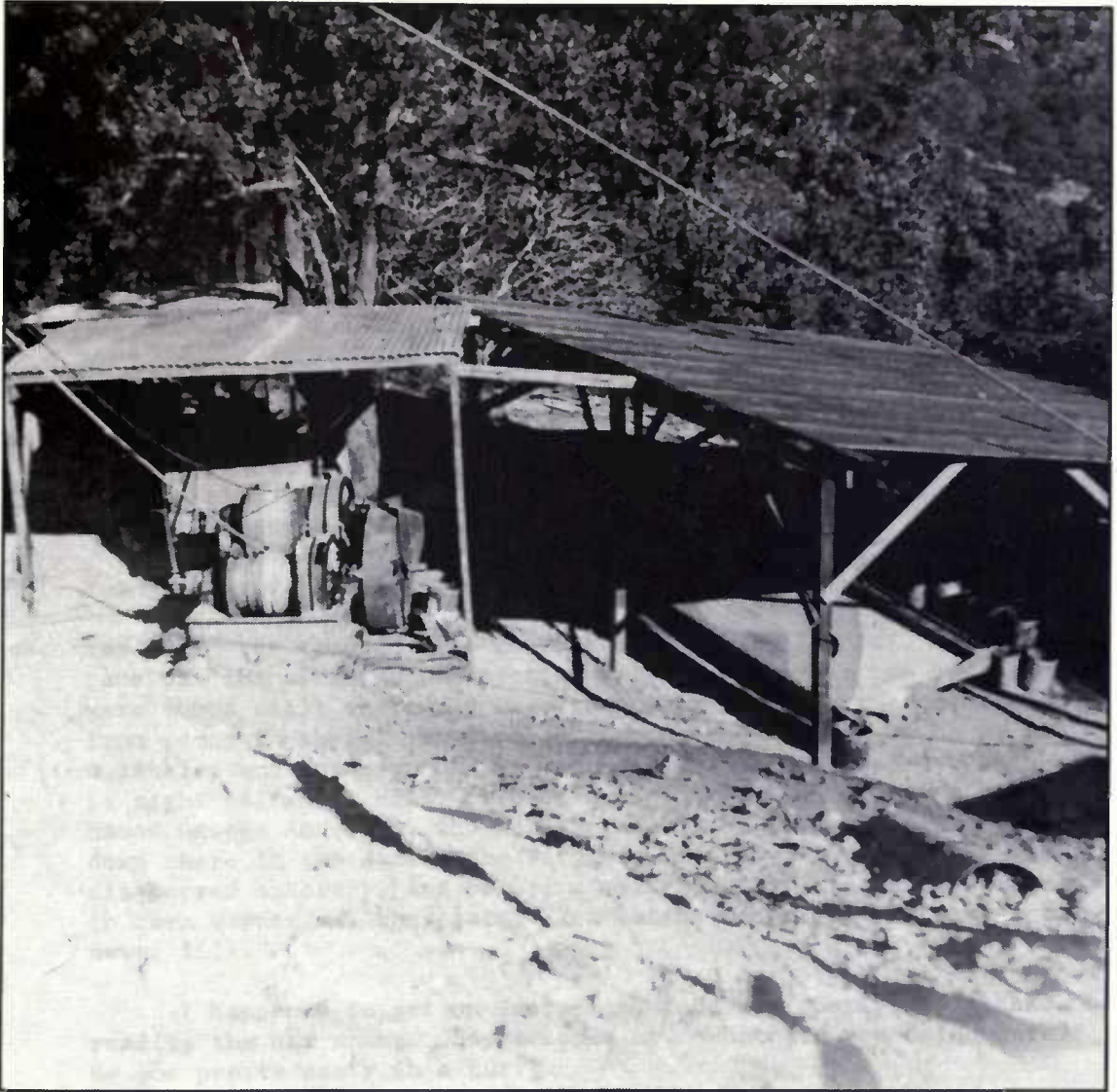
Anderson Plant at Oat Hill Mine.
