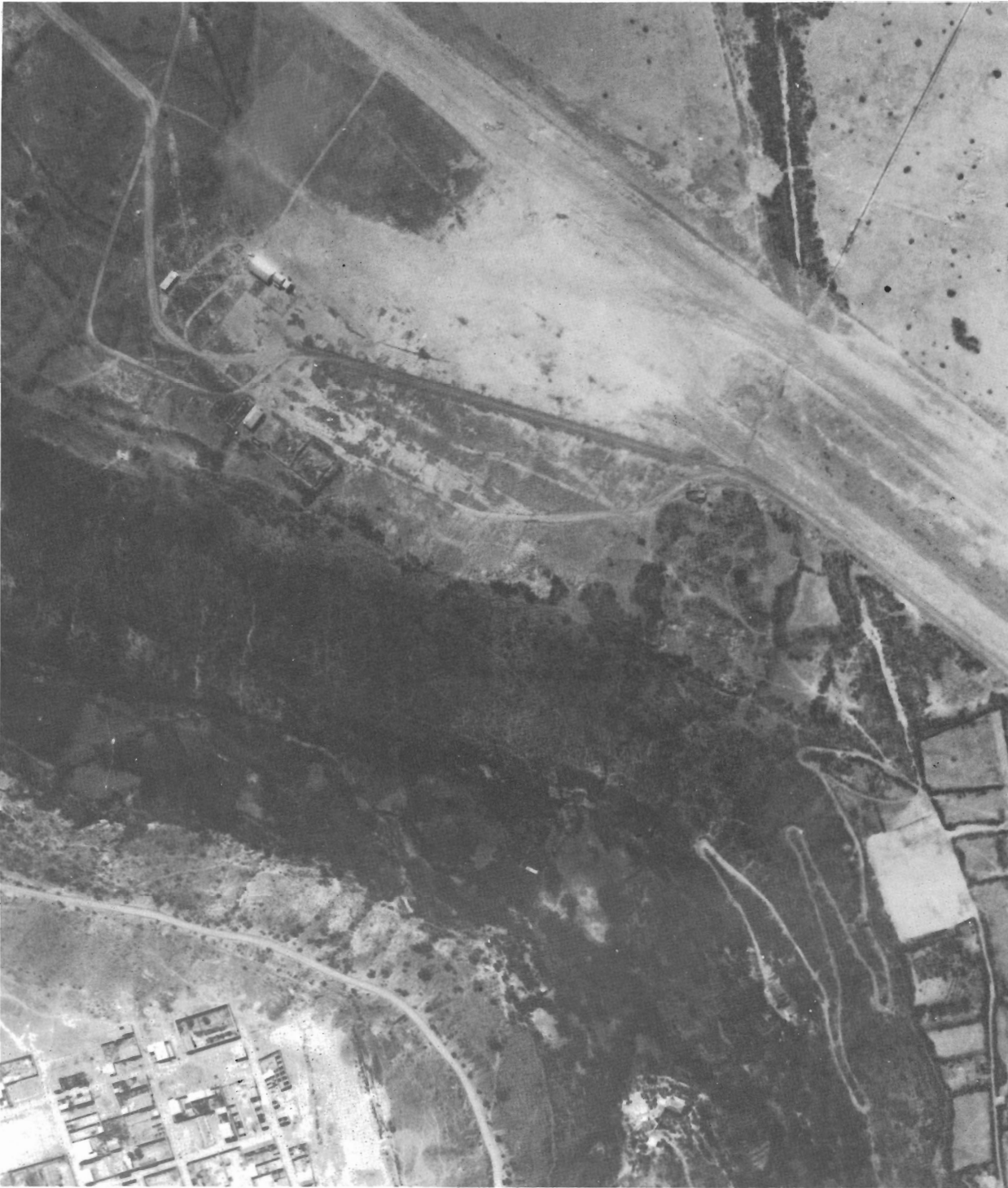
Fig. 7. 1970 aerial photograph of Conchopata, with Area A at center right. Lumbreras' 1970 building complex excavation appears as an elongated rectangle in the cleared, northwestern corner of Area A. Airport runway (oriented almost due north-south) and associated construction obliterated the Tomb X complex as well as Area C-2, and gravely damaged Areas A, B, and C-1. Following enlargement of the airport in 1974, a series of buildings has been erected on much of the site. See Key to Illustrations.
