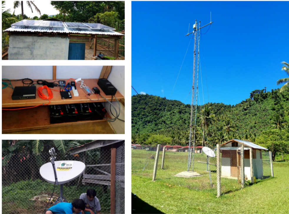
Figure 4.5: Components of a typical UP community cellular installation: solar panels (top left), battery bank and network hardware (middle left), VSAT antenna (bottom left), outdoor GSM radio system, tower and shelter (right).
