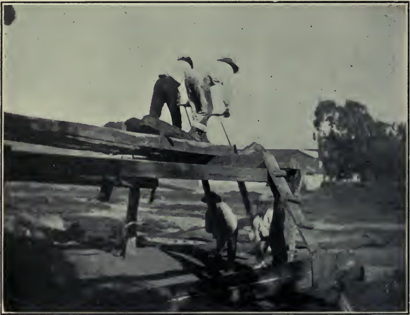
SAWING OUT BOARDS IN THE SHIP YARDS, CONSTITUCION.
