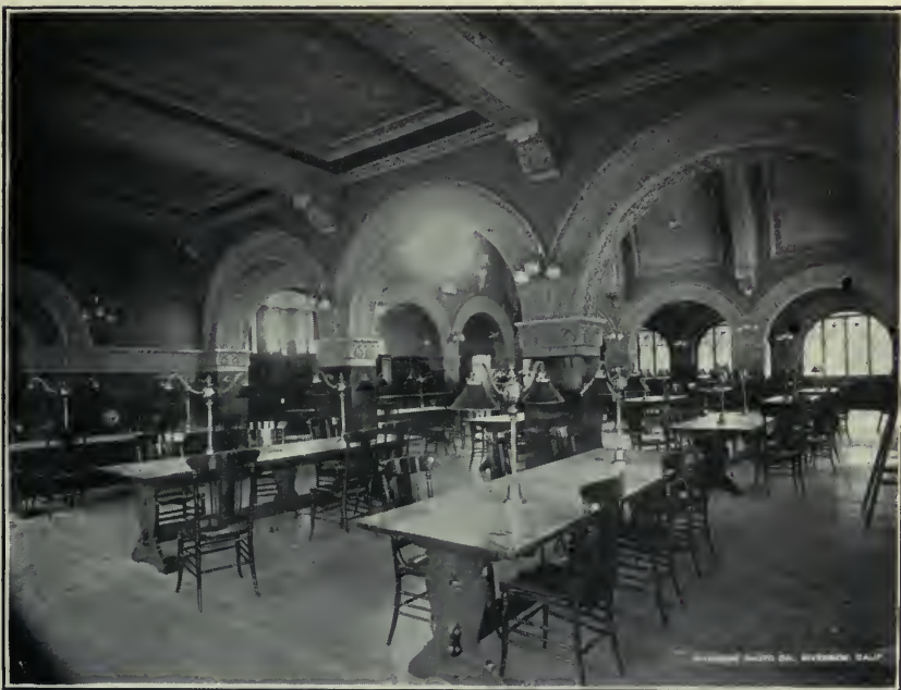
GENERAL INTERIOR, RIVERSIDE PUBLIC LIBRARY.
