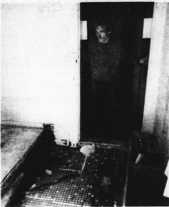
Steve Russell inspects a neglected shower area. (Photo: M. Hicks)
