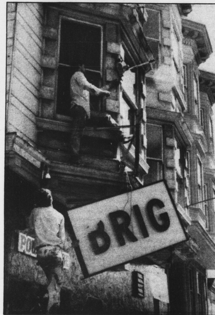
End of an era — The sign over the Brig comes down to make way for the Powerhouse, SofM's newest leather bar. (Photo: Marcus)
