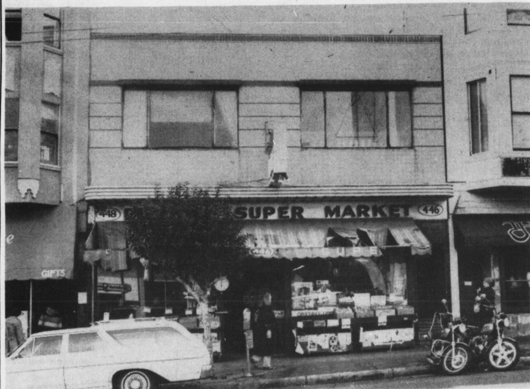
Castro Street site of new Atlas Savings and Loan branch. (Photo: Rink)
