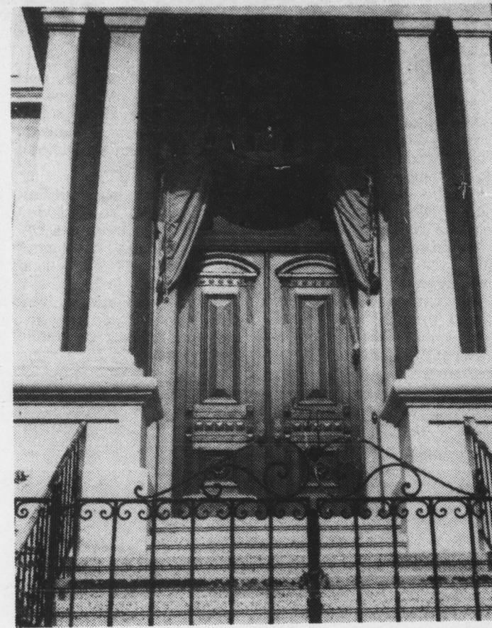
Pride Center entrance on Hayes Street — Hyatt Regency banquet nets $30,000 for million dollar renovation job and operating expenses. (Photo by Rink)
