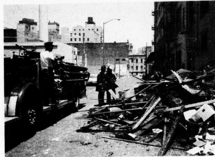
Surveying the damage.
