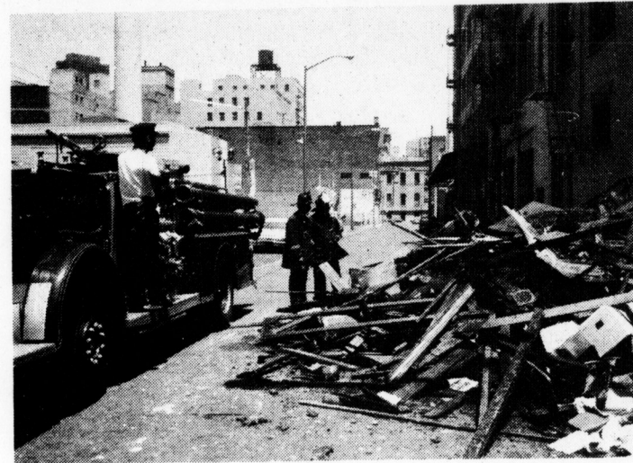
Surveying the damage.
