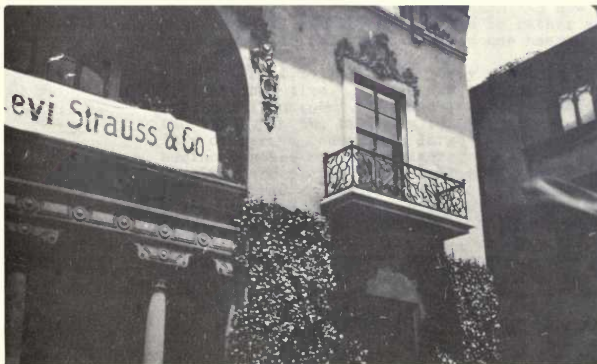
Home at 1666 Pacific Avenue, San Francisco Temporary headquarters for Levi Strauss & Co. after 1906 earthquake and fire.
