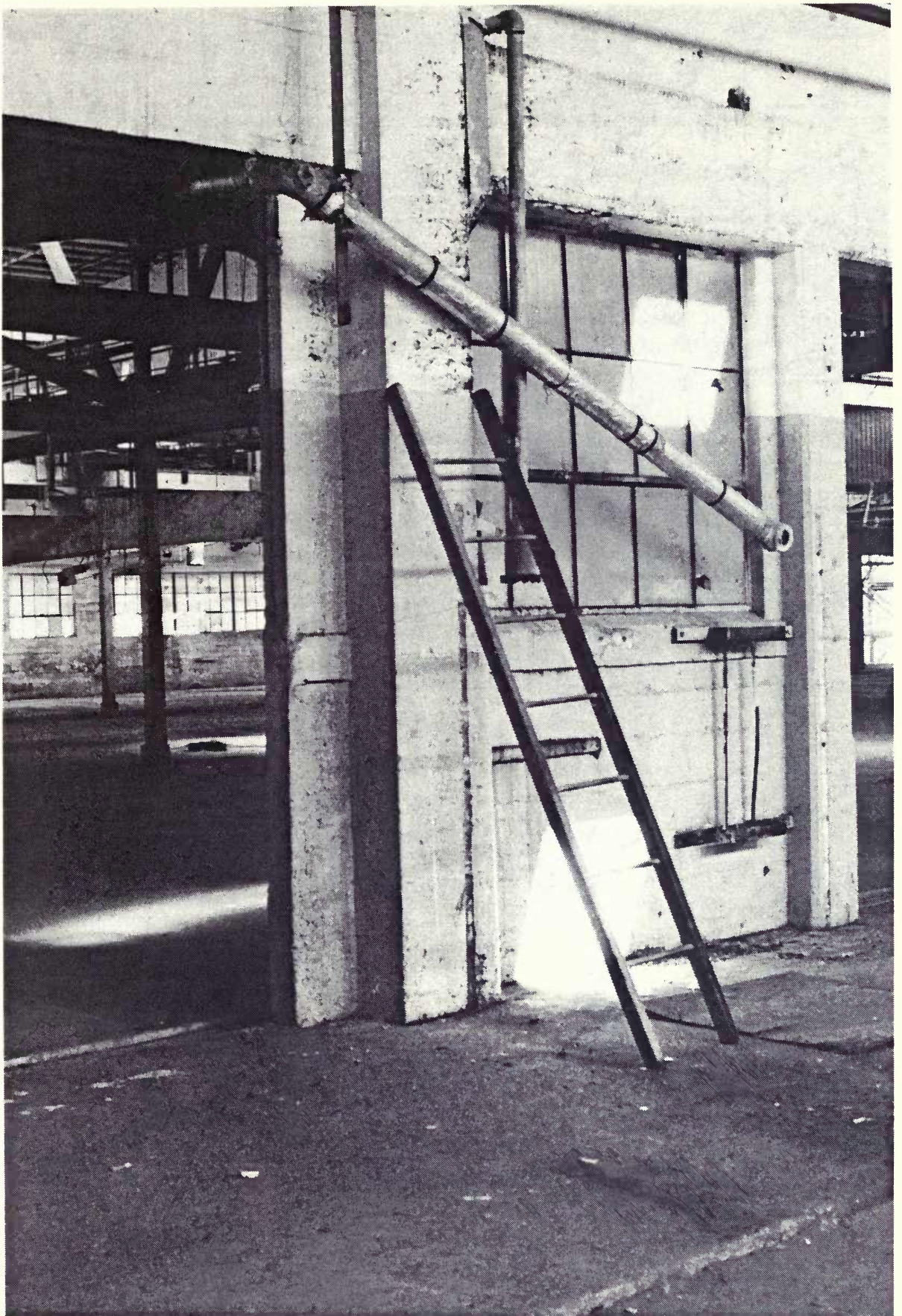
Interior of the former Filice & Perrelli Canning Company, in operation from 1930 to 1958. The building was sold to the California Cannery and Growers Association.
