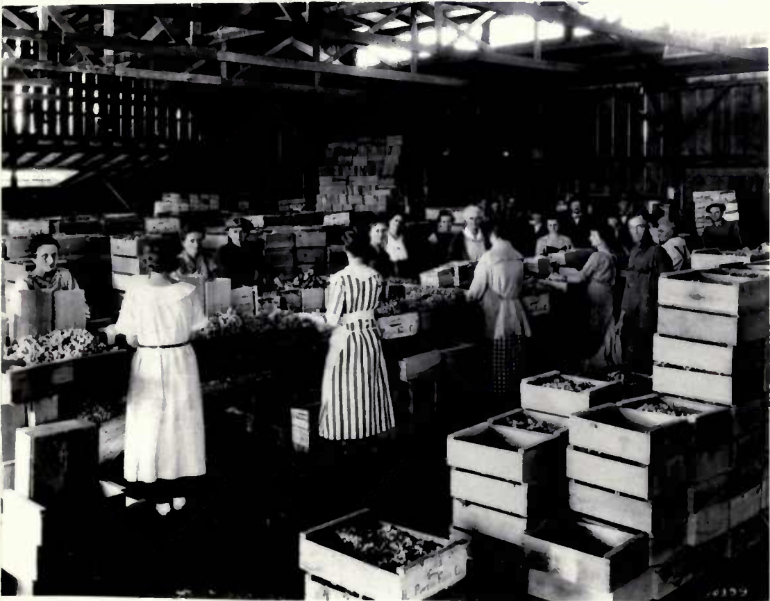
Powers Packing Sheds
