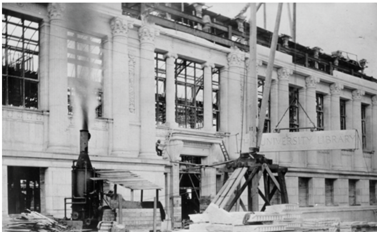
A 1909 photo showing the placement of the lintel and entablature over the north entrance to Doe Memorial Library.
