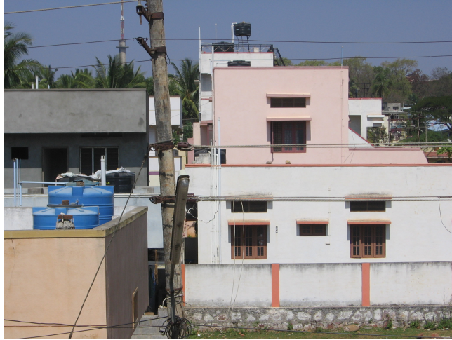
Figure 5-6 An Example of Storage Tanks on Roof Tops in Hubli-Dharwad
