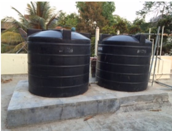
Tanks on a Two-Story Building Top
