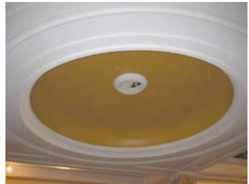
The gold-leaf dome progresses during construction.
