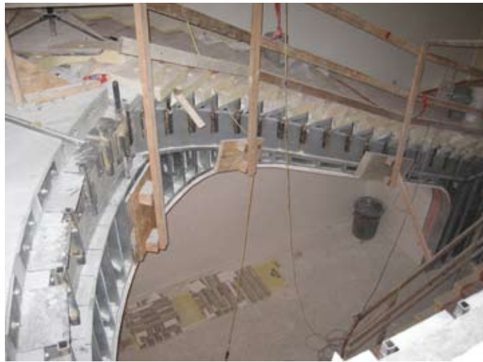
The grand staircase during construction.
