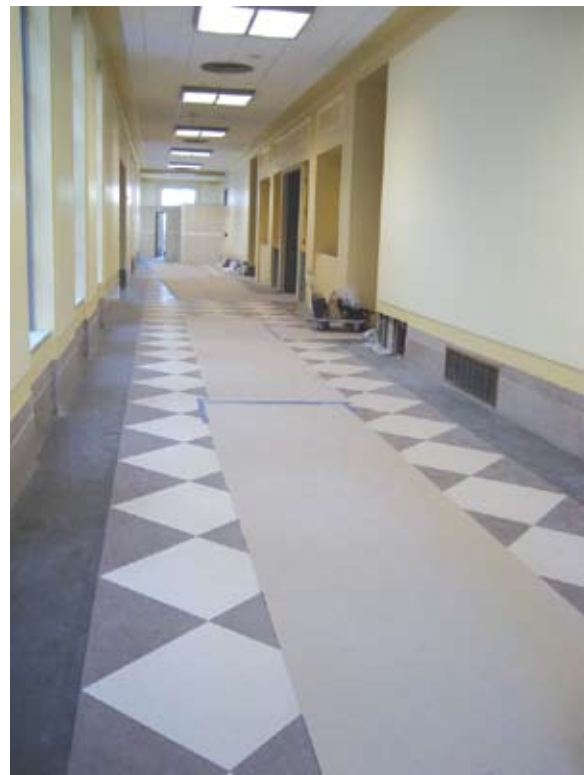
Public corridor between Doe and Doe Annex, 2nd floor.
