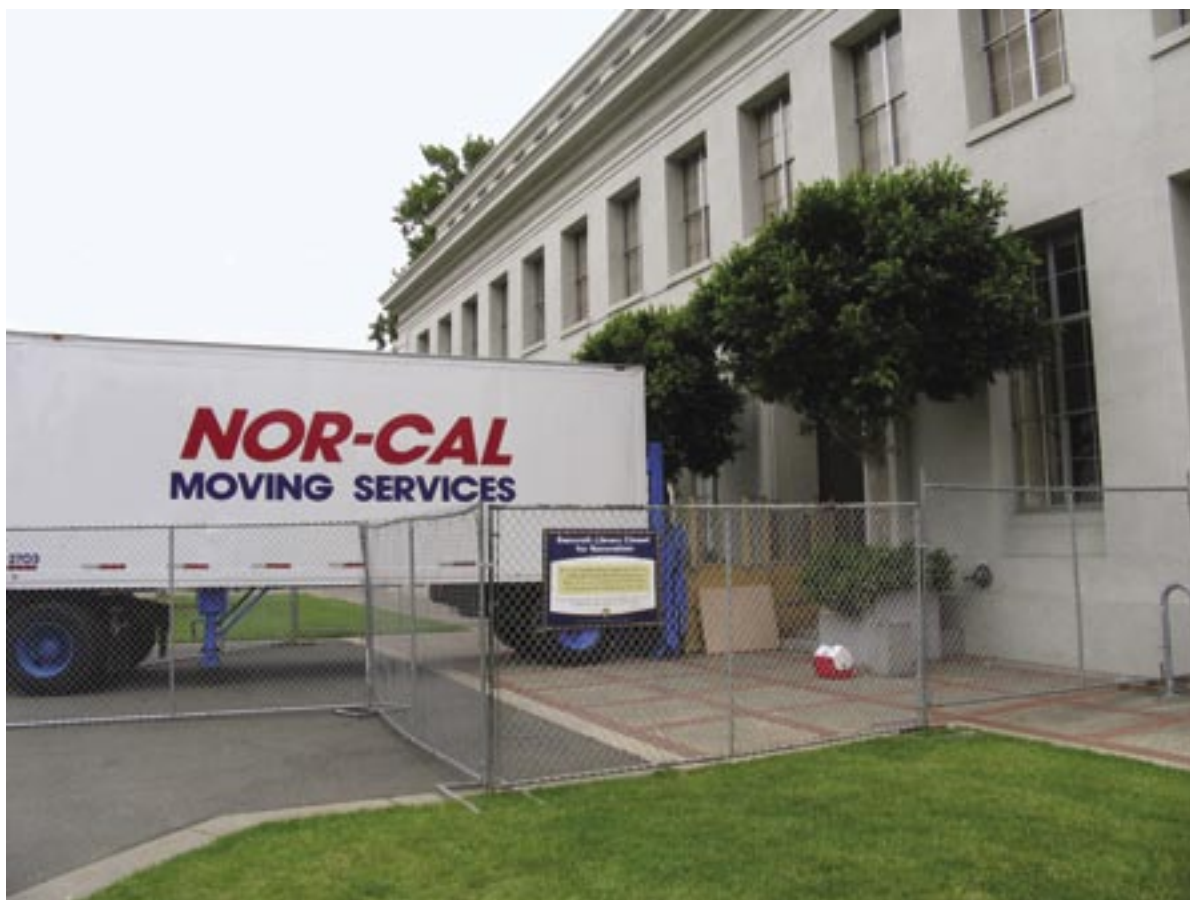
A temporary fence and specially built ramp were constructed to ensure safe transport to the Northern Regional Library Facility in Richmond.
